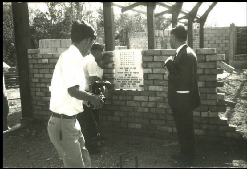
Laying the foundation stone for the new Rawang B-P Church, Muar, Malaysia
