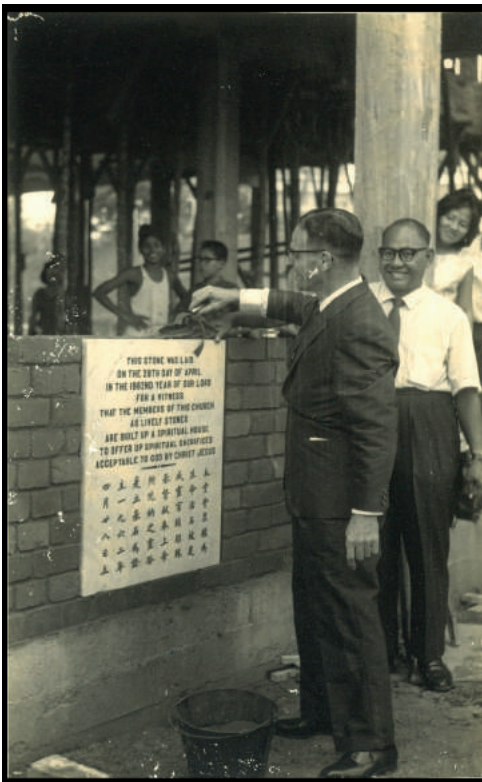
Paul Contento laying the foundation stone for Life B-P Church at Gilstead Road
