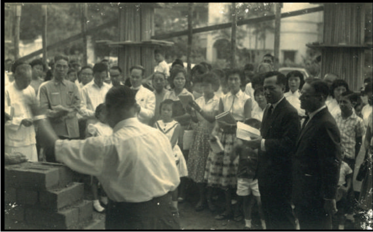
Speaking at the laying of the foundation stone for Life B-P Church at Gilstead Road, 28 April 1962
